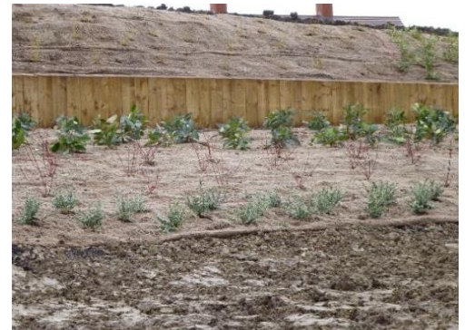
Use of a natural geosynthetic to control soil erosion and promote vegetation cover and landscaping
