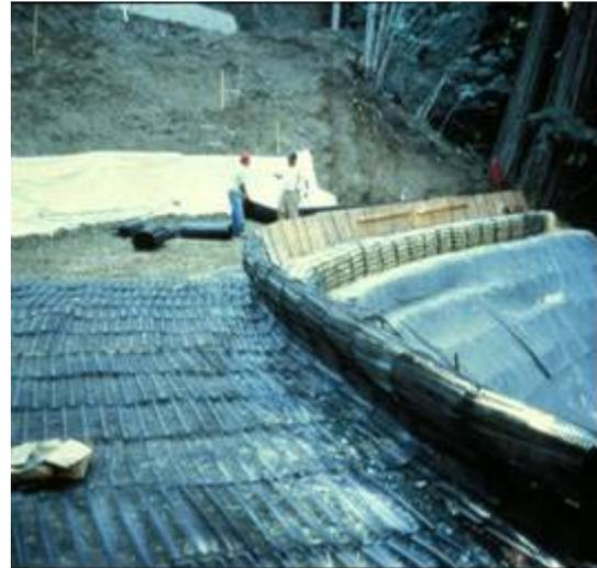
Example remediated slope with reinforced slope structure
