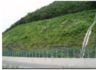
Completion of slope
