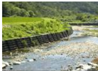
Completion of channel
