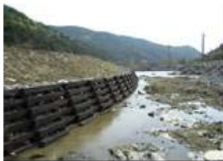
Construction of PE Block
