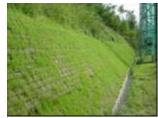
Completion of slope
