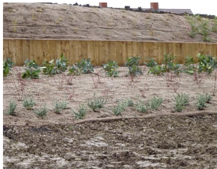
Use of a natural geosynthetic to control erosion and enhance vegetation
